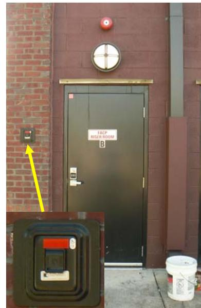
An exterior key vault has been installed beside a fire protection equipment room door to provide keys to firefighters for the facility.
