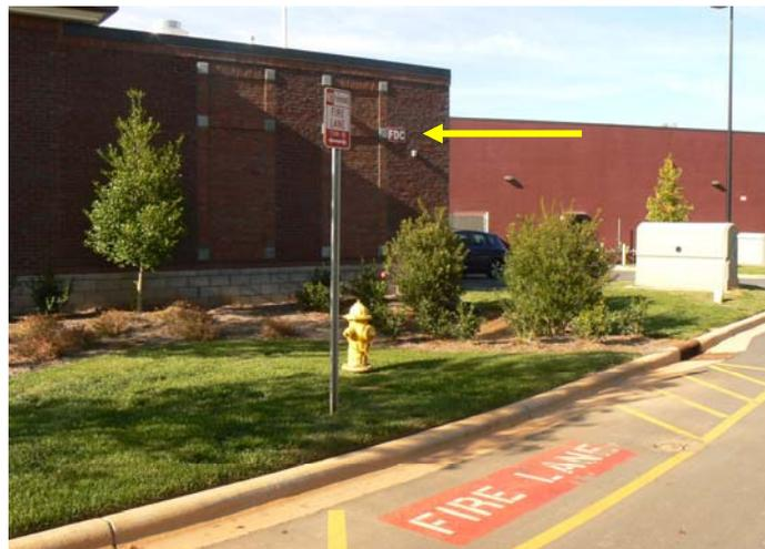
The line of site to the Fire Department Connection on this building is impeded by shrubbery. A "FDC" sign has been placed on the building to indicate the location.
