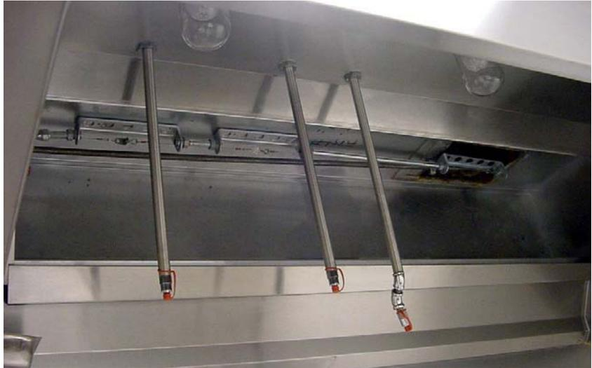
System Nozzles – Fusible Links (In Hood)
